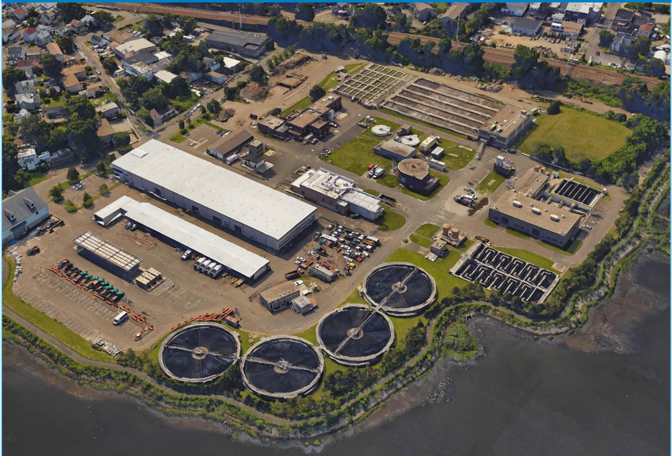
The Wastewater Treatment Plant at Liberty Point
