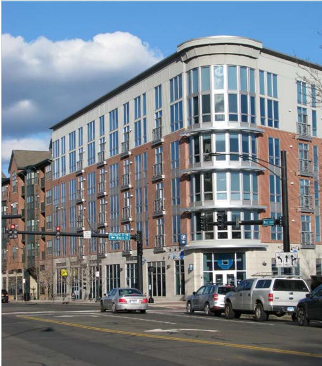
Waypointe is one of several recent multifamily developments providing greater housing choice
