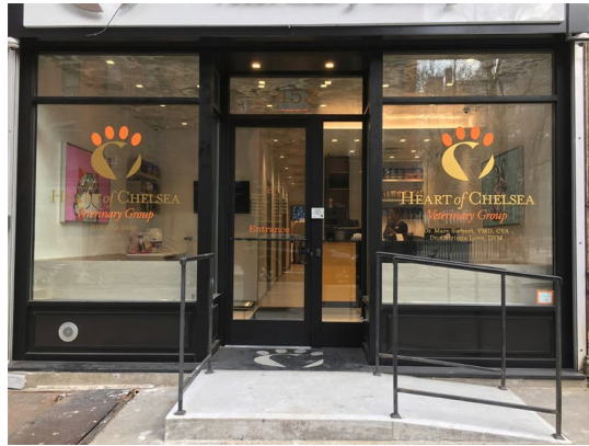
Figure 12: Contemporary Storefront Source: Skywindowsnj.com
