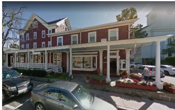
Figure 3B: Rockport, MA. Source: Google Street View
