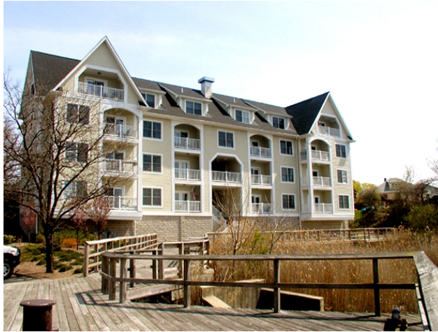
Figure 10: Residential Source: Unknown, provided by the City of Norwalk
