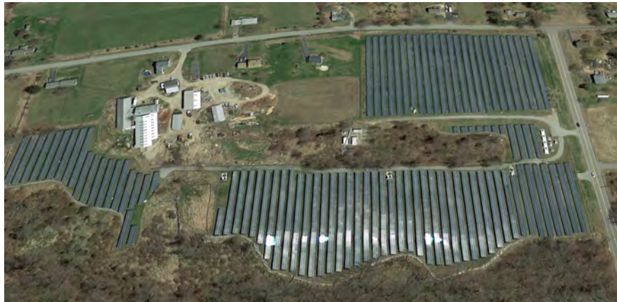
4.7 MW Mountain Ash Solar Farm and Battery Energy Storage, Norwich, CT
