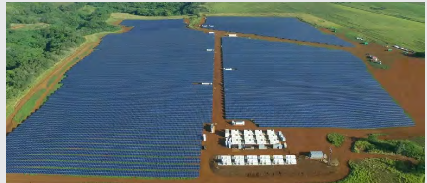
13 MW Tesla solar farm paired with 13 MW/ 52 MWh battery storage facility Kaua'i, Hawaii
