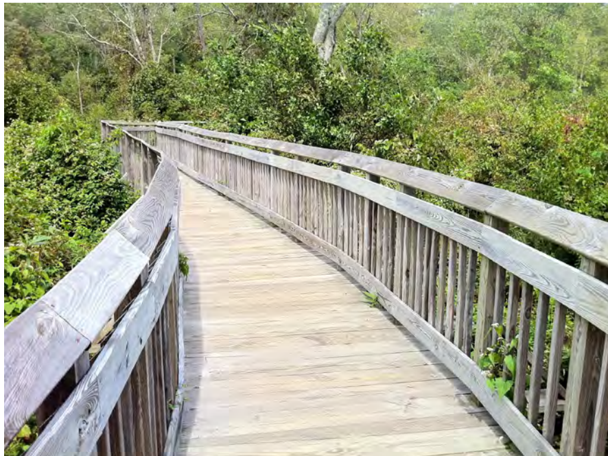
Areas of Manresa Island would likely require the construction of boardwalks to provide access to viewing areas. The example above is the Paul F. Wildermann Boardwalk, Chatfield Hollow State Park, Killingworth, CT Source: commons.wikimedia.org
