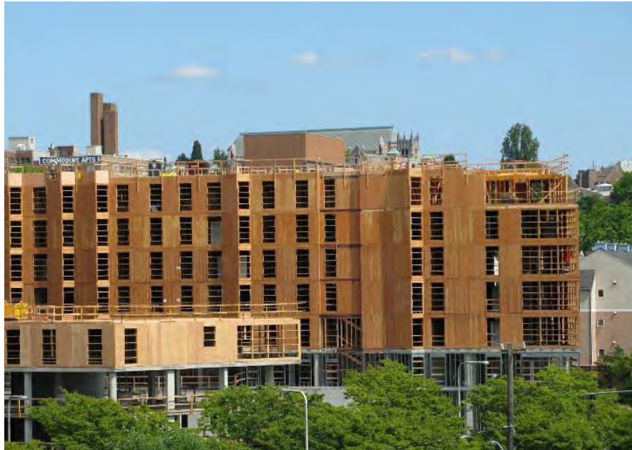
Example of Type IIIa construction: Five stories of wood frame construction over a concrete podium base.
