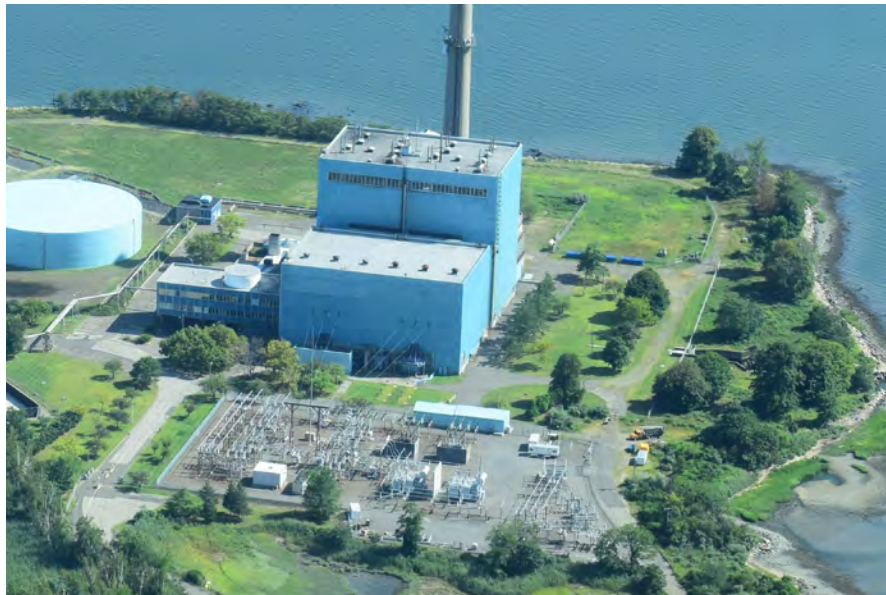
Eversource's electrical substation is immediately north of the power plant and connects to underwater transmission lines that travel across the Long Island Sound to the Northport Power Station in Long Island.
